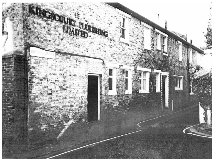
Fig. 2. The former Kingscourt Publishing Limited, 20, British Grove, Chiswick (now demolished), the site of Alpha & Omega Cottages.
